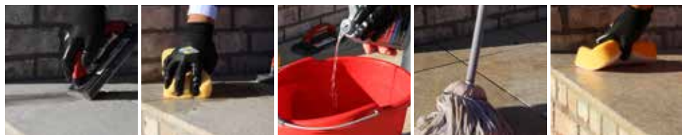
PIC 1. Fill joint with grout.
